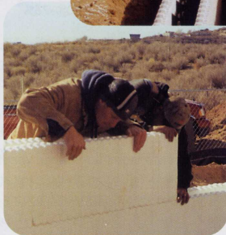
In addition to framing the Vision House, Earth Source Construction is the foundation sub as well. Above, Jeremy Schmidt (Shawn's brother) sets ICFs that will (below) create a perimeter wall.
