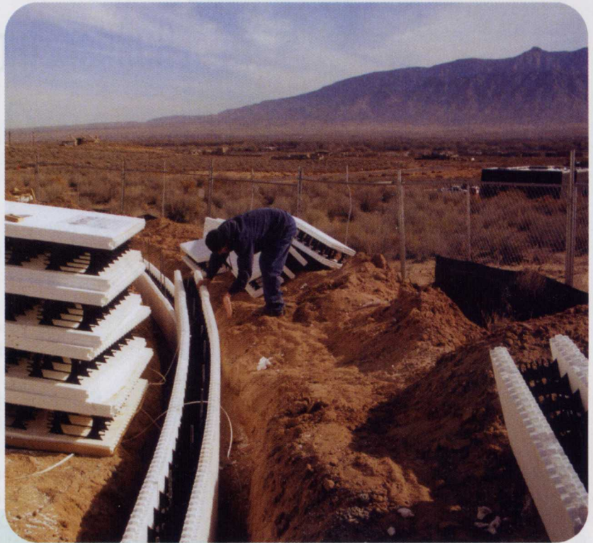
In addition to framing the Vision House, Earth Source Construction is the foundation sub as well. Above, Jeremy Schmidt (Shawn's brother) sets ICFs that will (below) create a perimeter wall.
